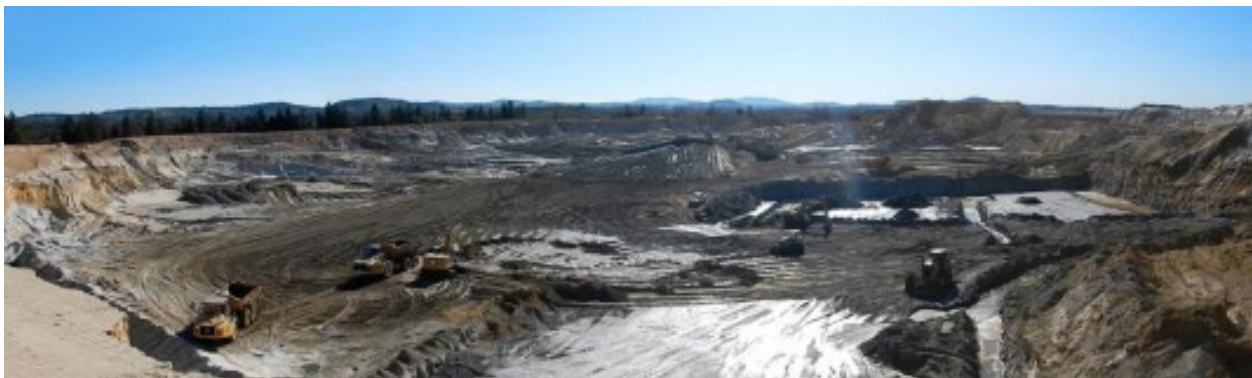
According to the California Water Quality Control Board, TPM is operating “a new unpermitted heavy mineral mining and processing operation,” shown above, in violation of California law. (© Central Valley Regional Water Quality Control Board)
